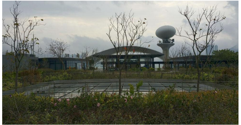
Rooftop Garden at Kai Tak Cruise Terminal
