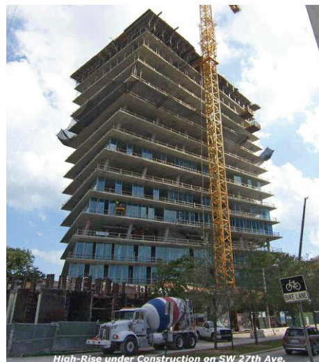
High-Rise under Construction on SW 27th Ave.
