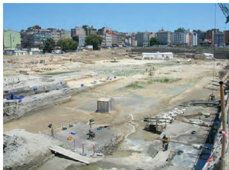
Some part of excavation site in Yenikapi
