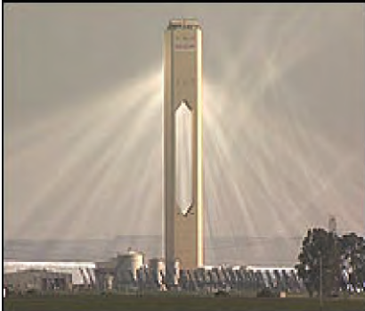
160 Steerable mirrors concentrate sunlight on the boiler 115 m high boiler tower
