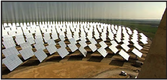
160 Steerable mirrors concentrate sunlight on the boiler 115 m high boiler tower
