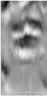
Baird's first pictures 1926 using 30 lines
